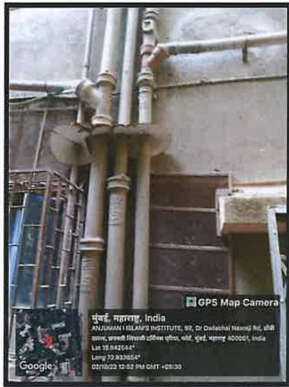
Pipes Carrying Water
