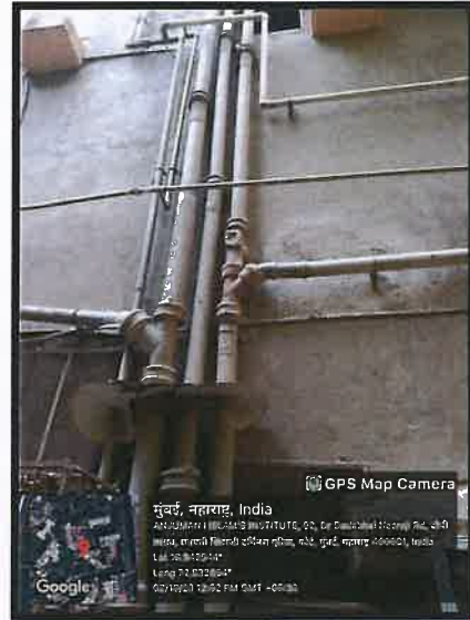
Pipes Carrying Water
