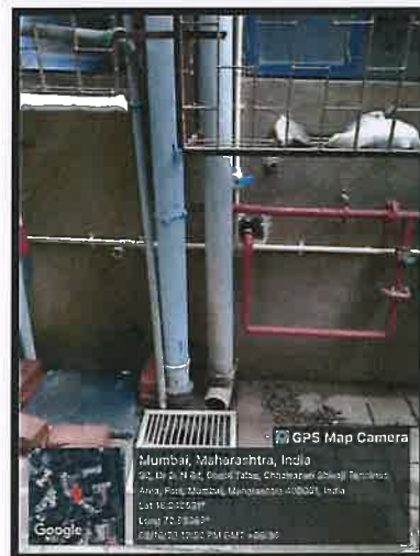
Sewage Pipes disposing the waste water in seepage tank
