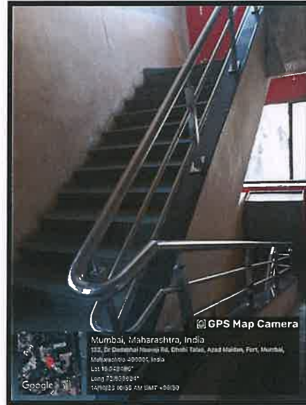
Railings alongside staircase
