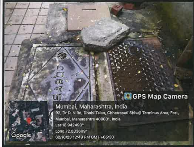
Drainage & sewer ducts
