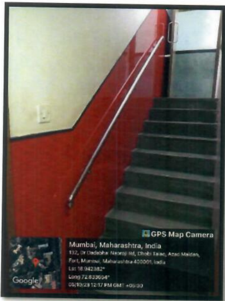
Railings alongside staircase
