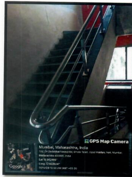
Railings alongside staircase
