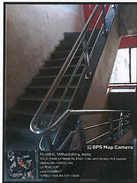
Railings alongside staircase
